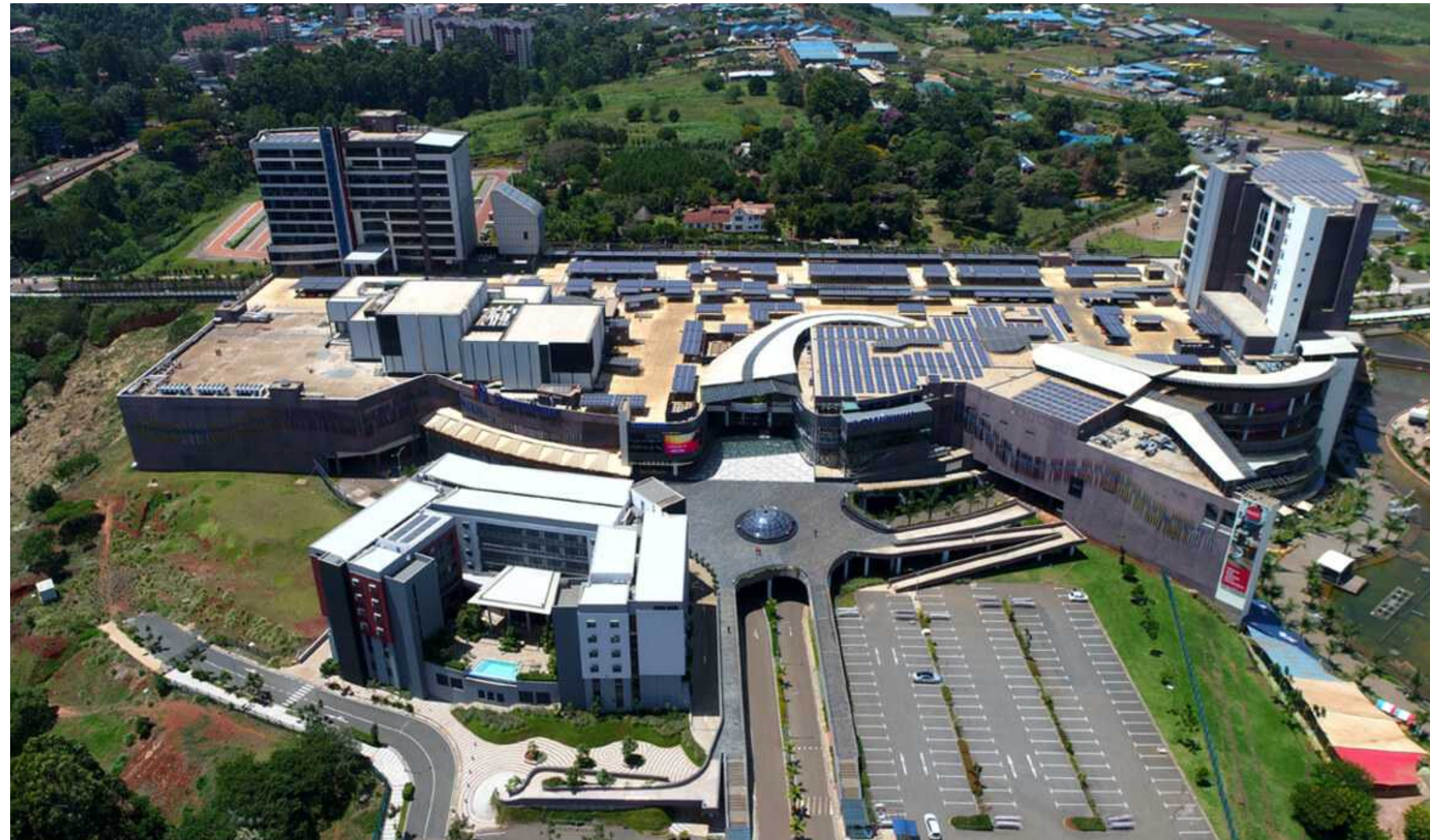
Rooftop Solar farm
