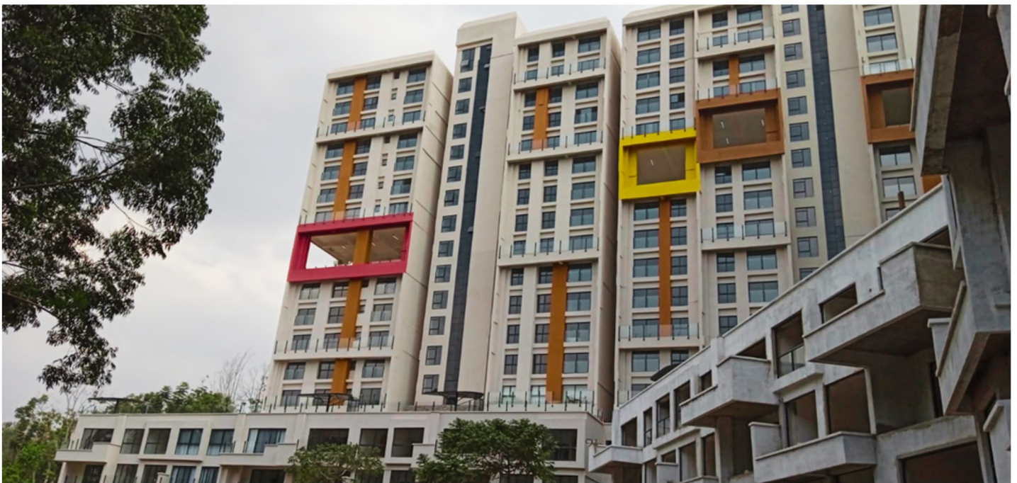
Phase 1 (Block D & E)
