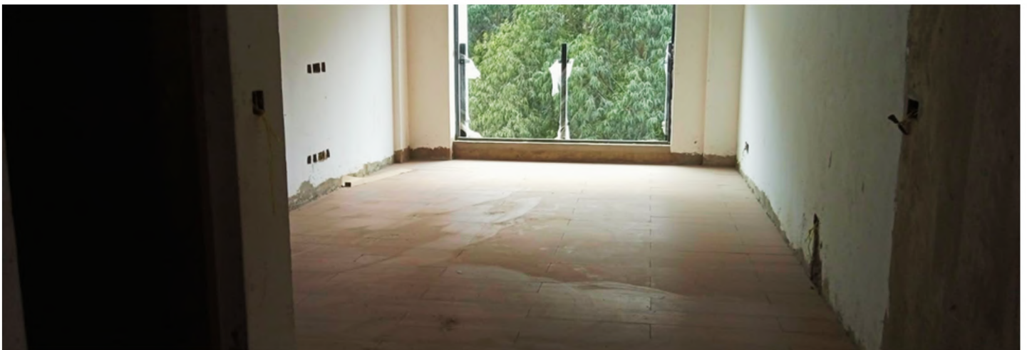
Tiling at level 8
