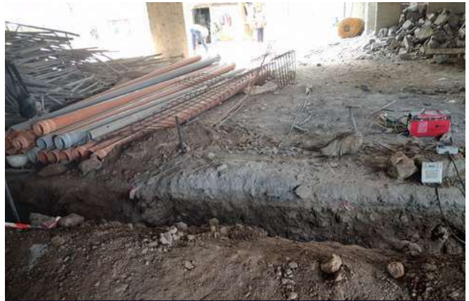
Sewerline and Boundary wall Installation
