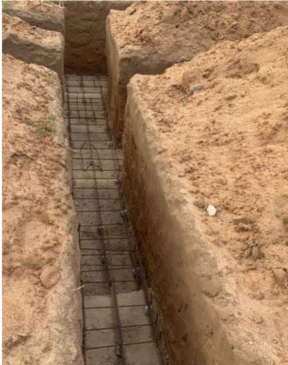
Fixing of Reinforcements in foundations
