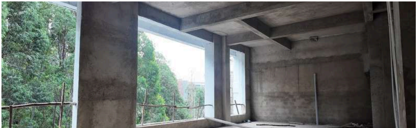
Open Garden Plastering
