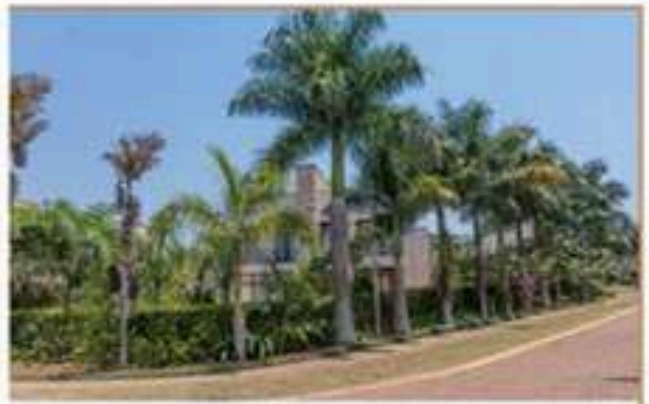
Paved roads & green Spaces
