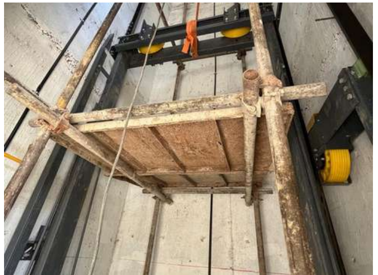
Lift Installation
