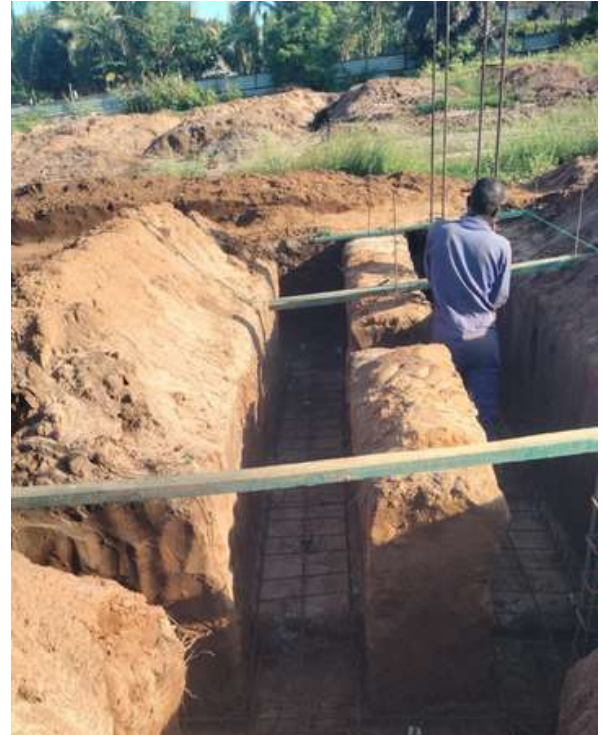
Fixing of Reinforcements in foundations
