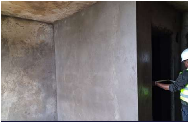
Plastering Block A
